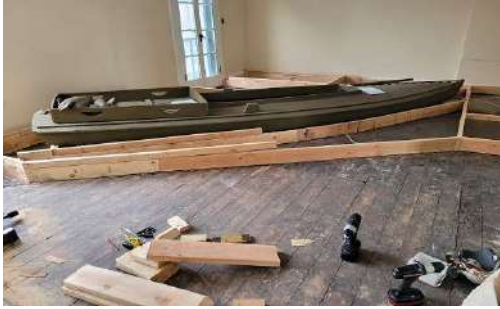
Left: Laying out the framework for the platforms
