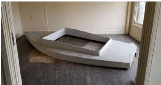
Left: Repaired south room with scooter
