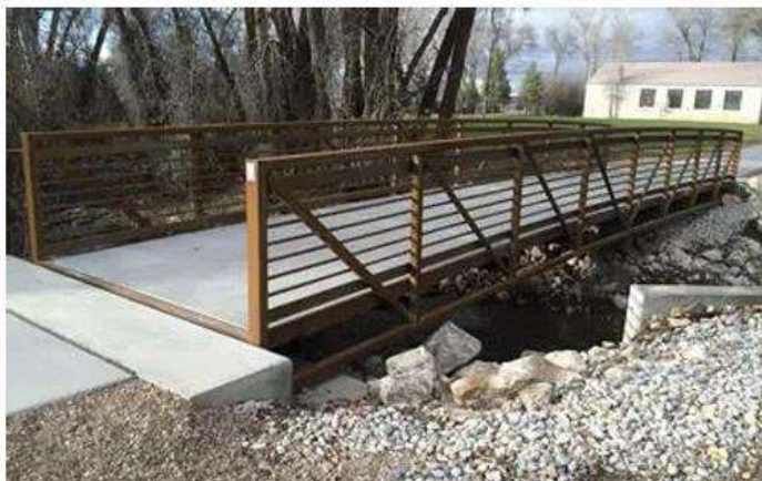
Manufacturer – CONTECH 8' x 10' truss bridge of weathered steel
