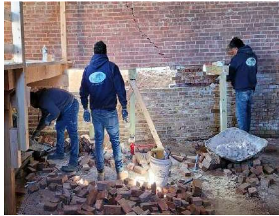
Working on the wall
